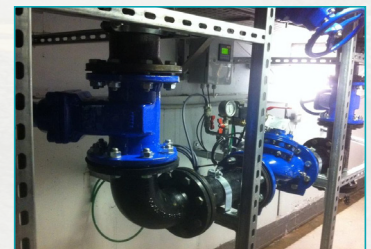
PRV Installation
