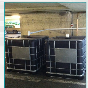
Water is held pending use in the tanks shown below.
